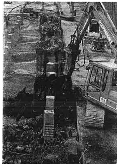
Photo 2: Hydraulic hammer mounted on a crane truck
